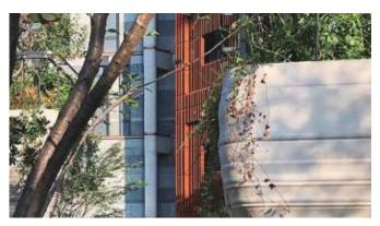
The pillar form is complex and traditional construction methods are not suitable in terms of feasibility and cost. The project team used **3D printing technology** to produce fiberglass-reinforced concrete materials and a corrugated coating on the surface of the pillars, with a facade effect that looks like sedimentary rock.
