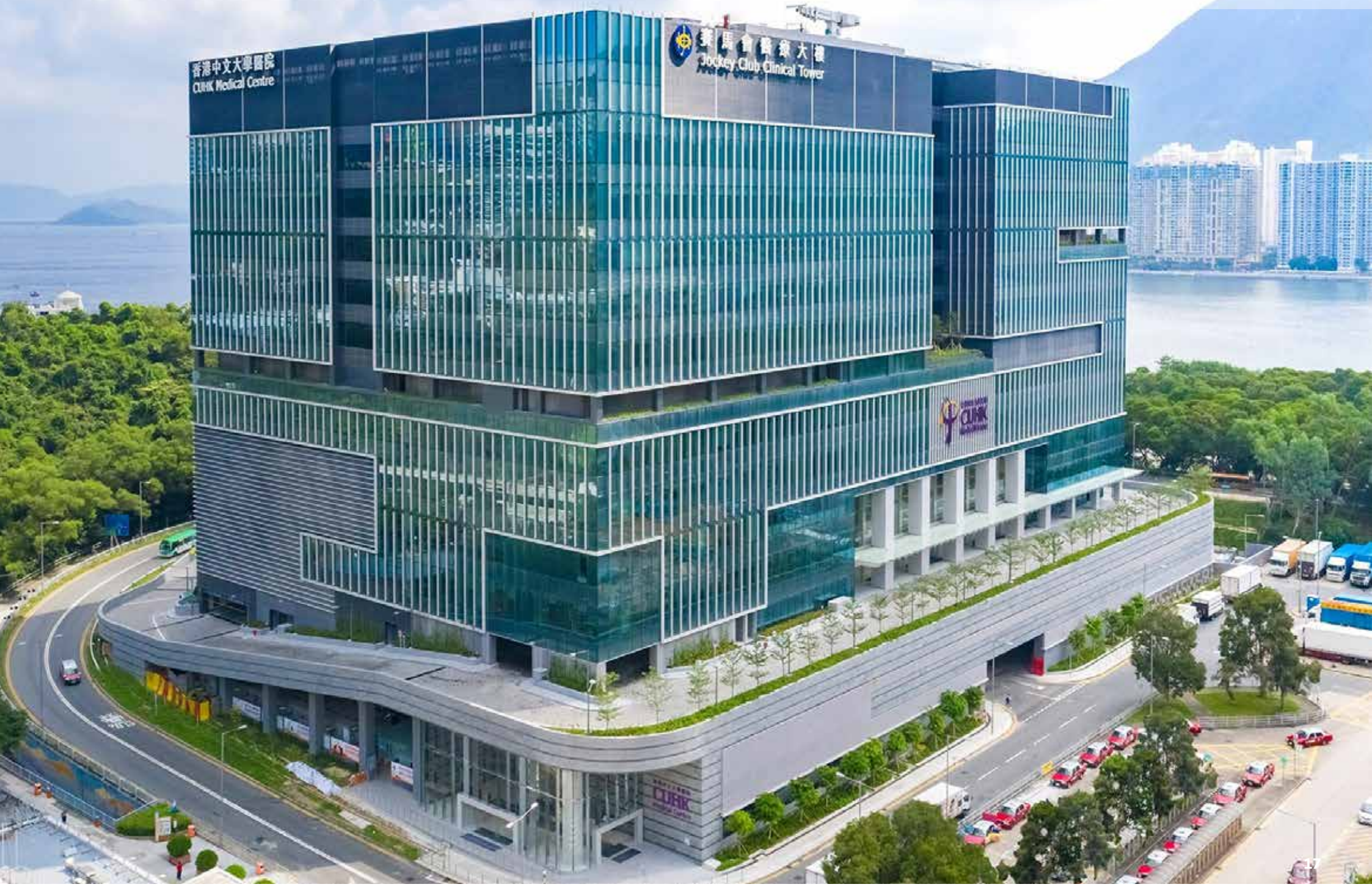
CUHK Medical Centre, Hong Kong
